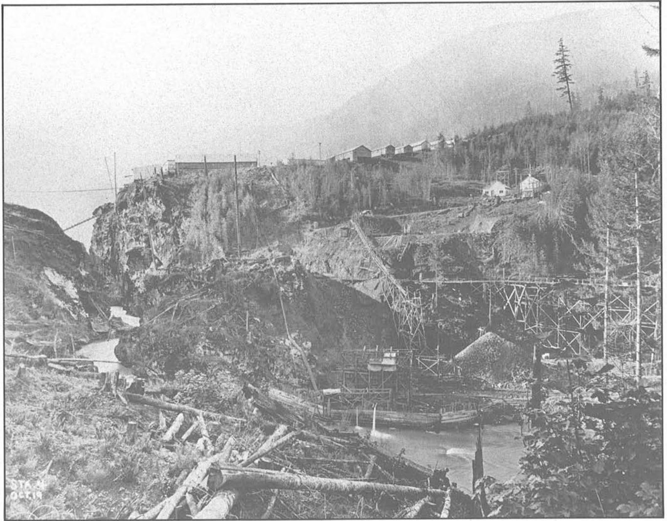
Glines Canyon project with power house in right foreground and dam in left background, October 19, 1926. (Northwestern Power & Light Company photo)
