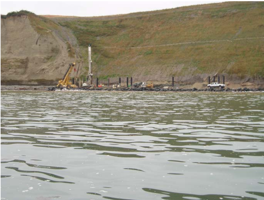
Port Angeles land fill closure project July 2007.
