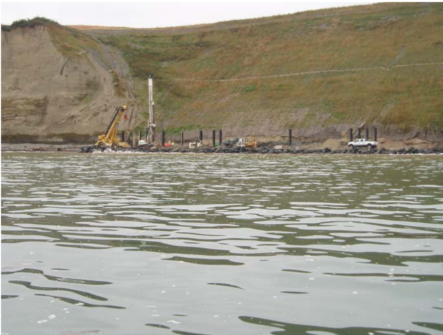
Port Angeles land fill closure project July 2008.
